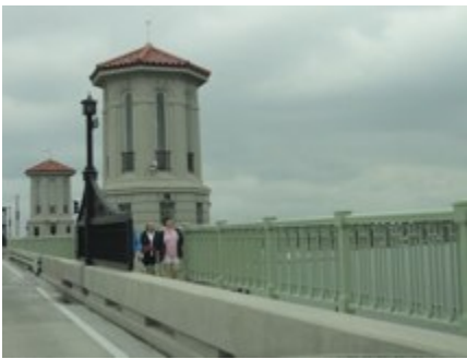
SALB Bridge walkers
