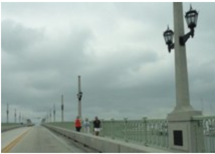
SALB Bridge walkers
